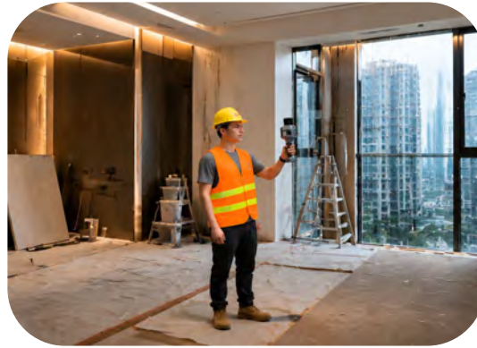
Interior Design and Refurbishment
